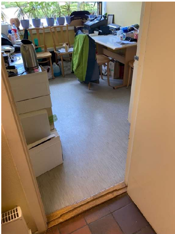
Figur 96 Linoleumgolv i lunchrum/pentry.
