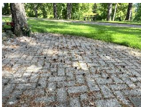
Betongmarksten i minneslunden
