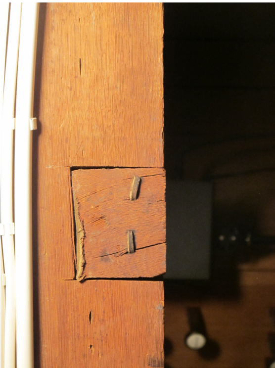
15. Traces of double imposts in the back of the RP case (north side)
