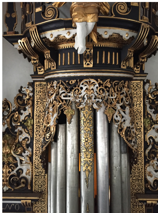
18. deformed pipe shades due to subsidence of the tower cap
