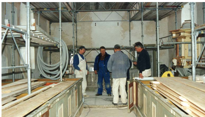
Håkantorps kyrka under renovering.
